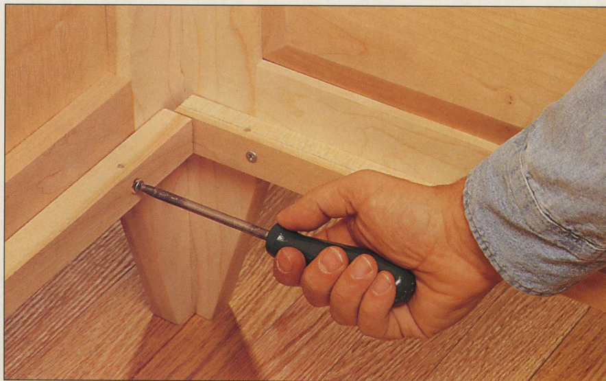
A ledger strip is fastened to the back bottom rail of a pie safe. Once strips have been attached to all four bottom rails, the bottom panel will be screwed to the top edge of the strips.
